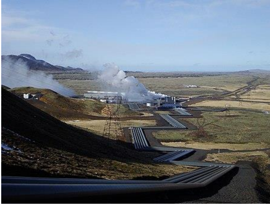
Hellisheidi Power Station, the third largest geothermal power station at ۳۰۳ واط
