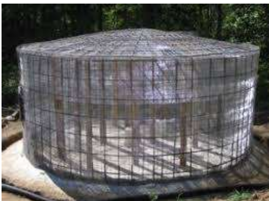
Fig.2. 5 — Ferrocement tanks for rain water collection
