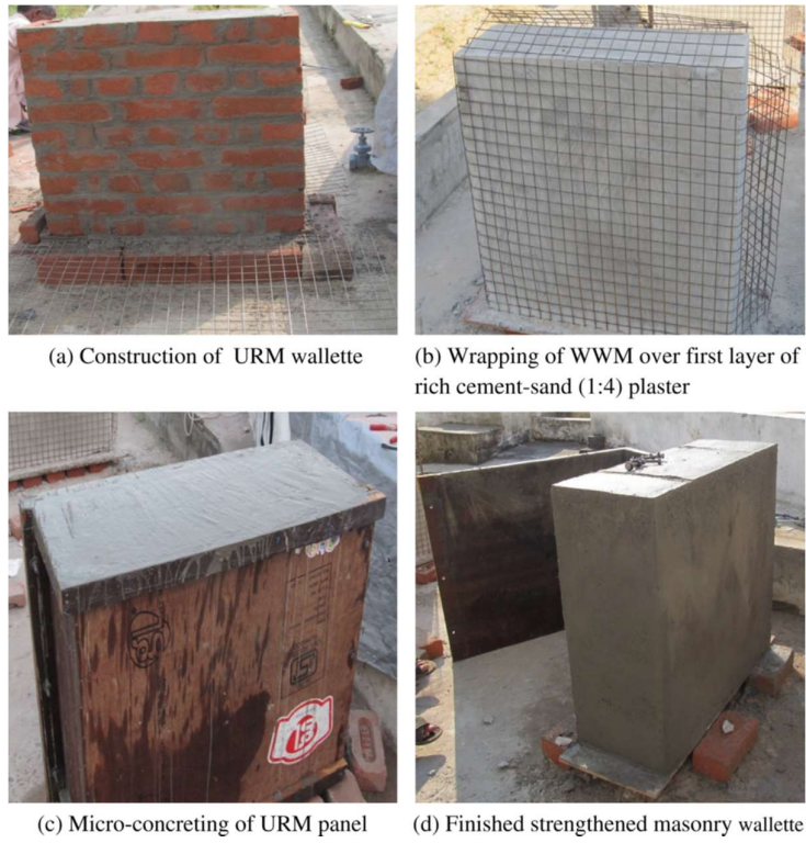
Fig.2. 11- Strengthening using ferrocement
