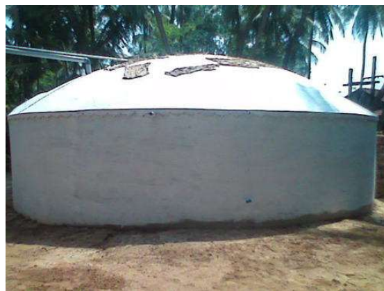
Fig.2. 6 —Rain-water ferrocement tank in India
