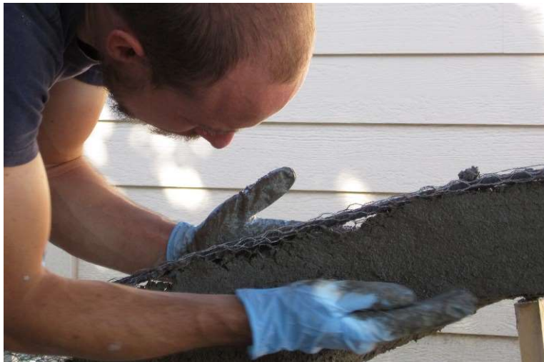
Fig.2. 18 -Spooner's deck bridge (while plastering).
