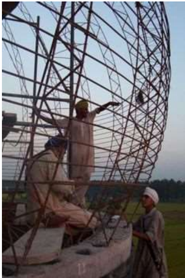
Fig.2. 4 —Ferrocement silos in India (under construction
