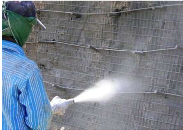
Fig.1. 1Wire mesh covered by mortar using shotcreteing to form a shell.
