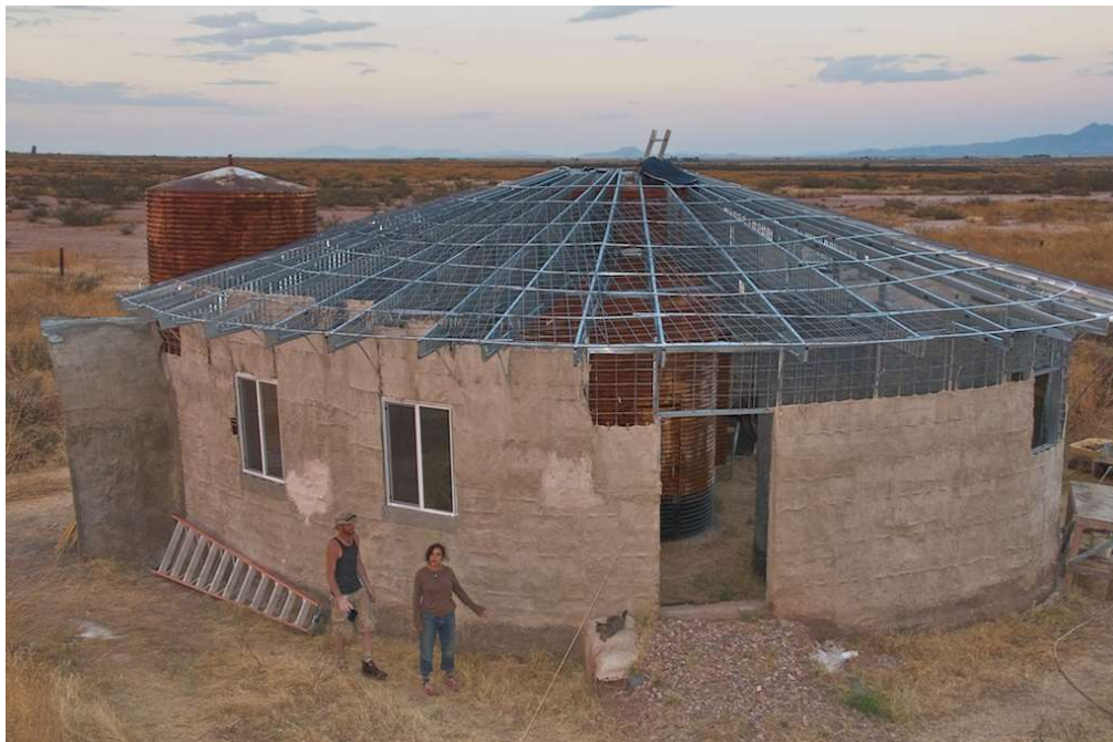
Fig.2. 9- Conical ferrocement roof
