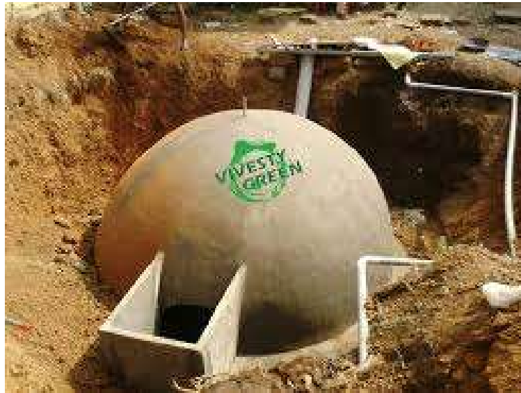
Fig.2. 15 - Ferro-cement biogas digesters completed
