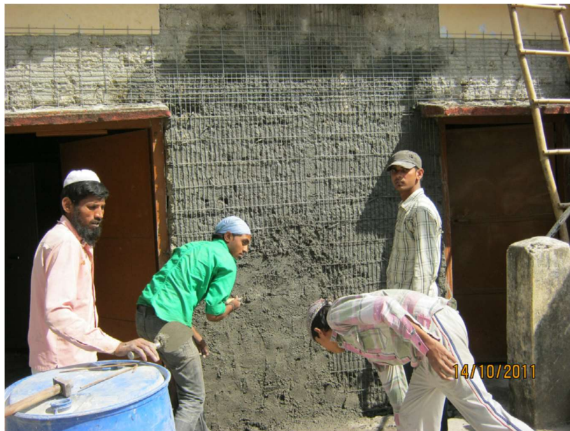
Fig.2. 10 - Strengthening using ferrocement in India
