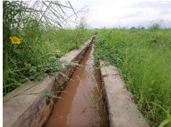
Masonry retaining wall canal (Msagali, Mpwawa, Central)
