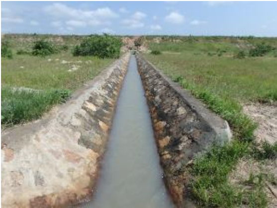
Masonry lining canal (Inara, Sikonge, Tabora)
