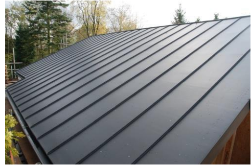
Figure 240, Zinc standing seam roofing.
