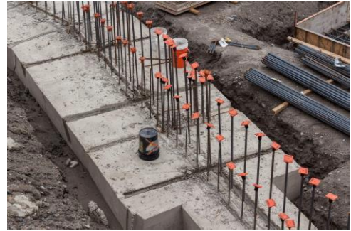
Figure 241, Cast-in-place concrete footing. Dylan Brown
