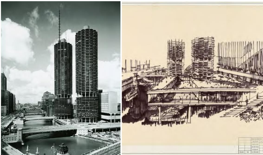
Fig. 1 –Marina City photographic image and sketch by Bertrand Goldberg (courtesy of the Art Institute of Chicago).
