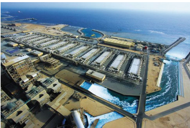
Fig. 16 Illustrates desalination plant in Saudi Arabia
