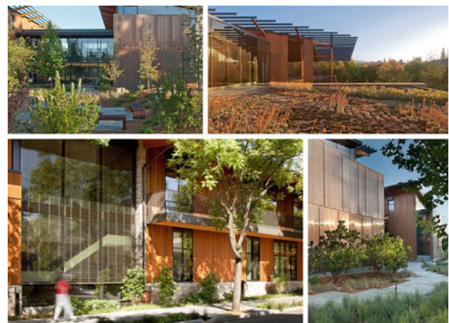
Fig. 2 The David & Lucile Packard Foundation Headquarters. American Institute of Architects (n.d.). Retrieved from: https://www.iaiatopten.org/node/403
