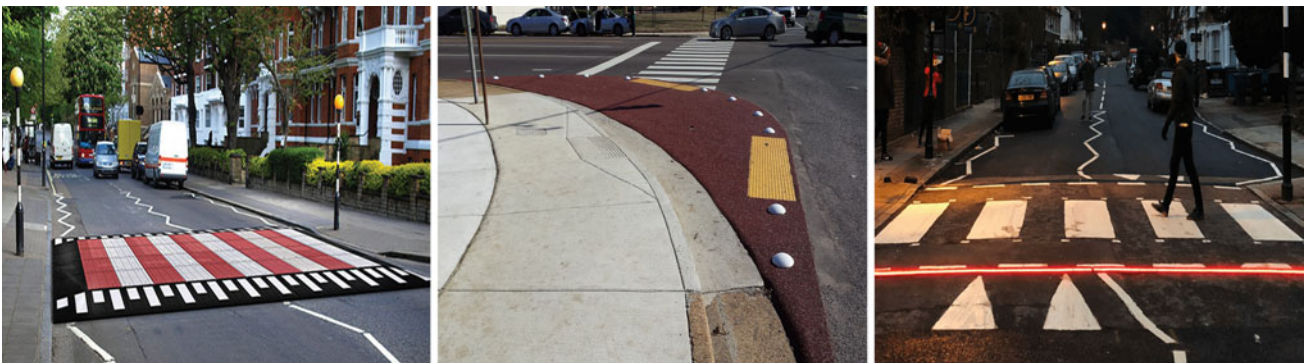
Fig. 10 Feasible traffic calming facilities
