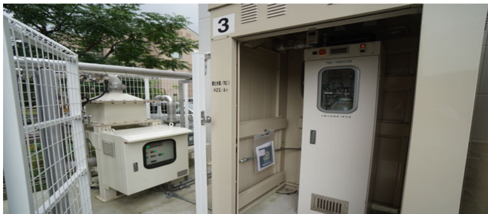
Fig. 5 Toxic gas management system
