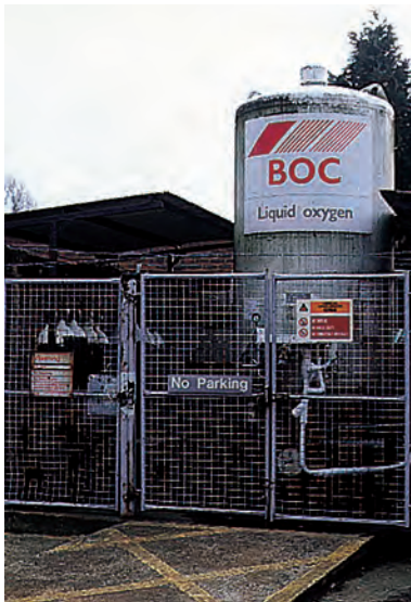
Fig. 1.18 A vacuum-insulated evaporator (VIE).
