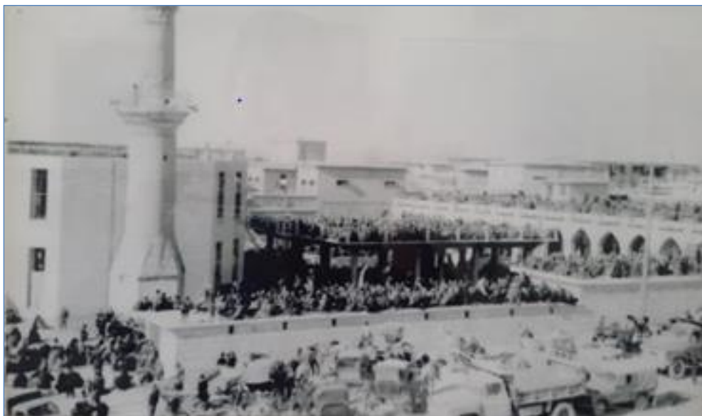
Fig. 3 : Elevation of the Mosque before Renovation. (Source: Awqaf archive)
