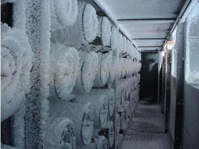
Cartridge Filters with Frost Build-Up Due to Cooling Tower Drift (Courtesy of Camfil Farr)
