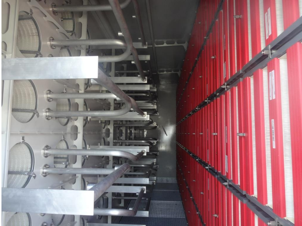
Al-Rasheed power plant/Baghdad/Iraq inside the filter house (the clean area)
