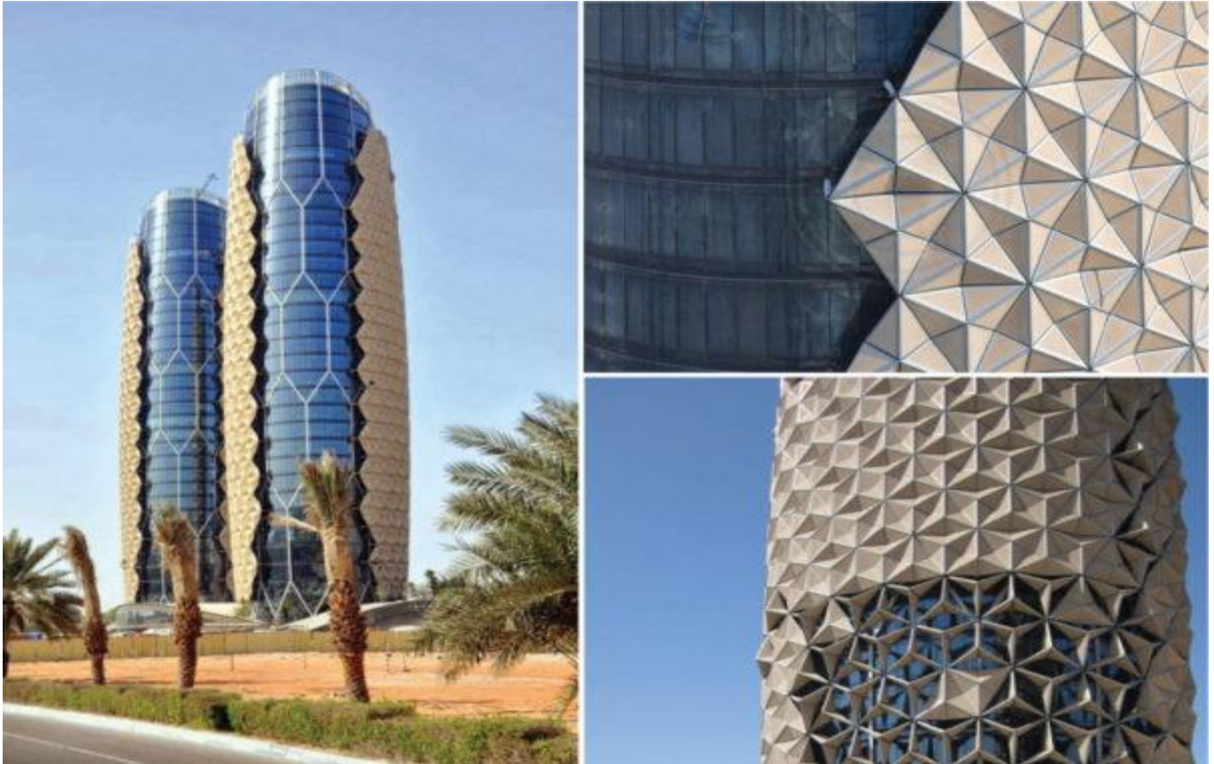
Al Bahar Towers Responsive Facade | Aedas
