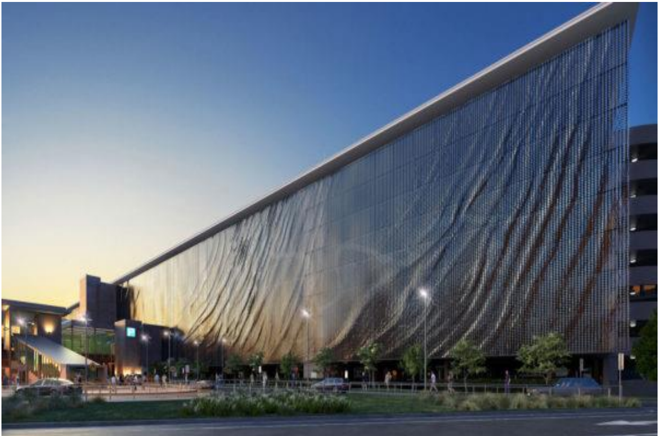
Brisbane Domestic Terminal Carpark in Australia | UAP
