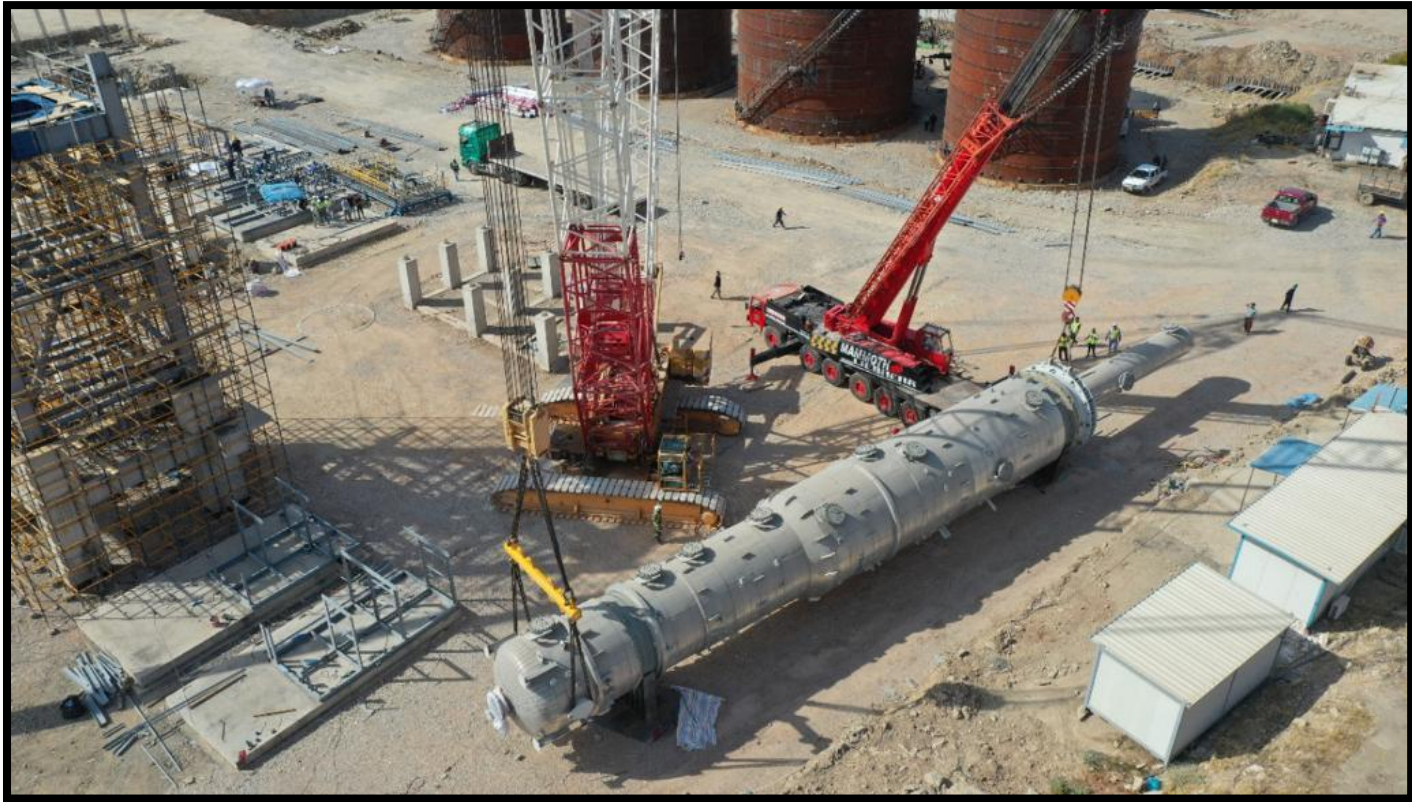
Figure 7,8 and 9: Pressure vessel during erection at site capacity 1400 MT per day
