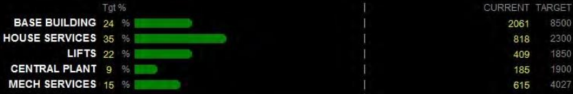
Energy Consumption for Today kWhrs
