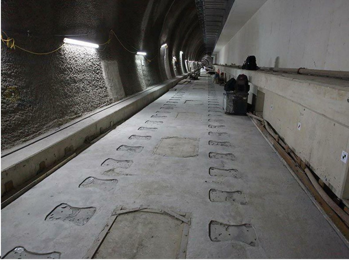
Figure (3) high strength Concrete
