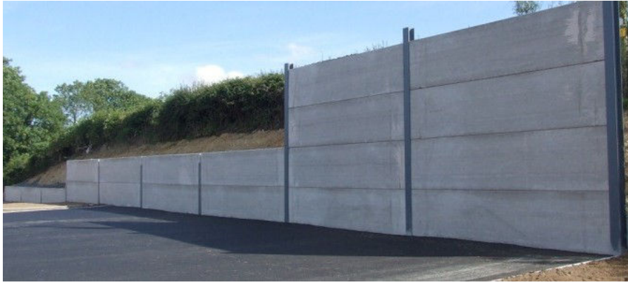
Fig. ٨٠ Precast concrete Fence
