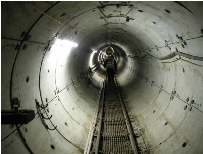
Fig. 20 Tunnel covered using Precast Concrete segments
