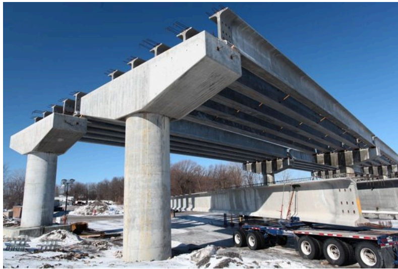
Fig. ١٣ Girder Bridge under construction
