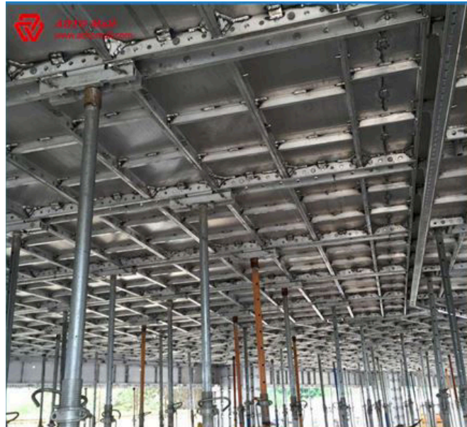
Fig. 4 Aluminum mould made by (ADTO Industrial Group) company in China
