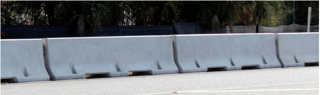
Fig. 20 Precast concrete barriers
