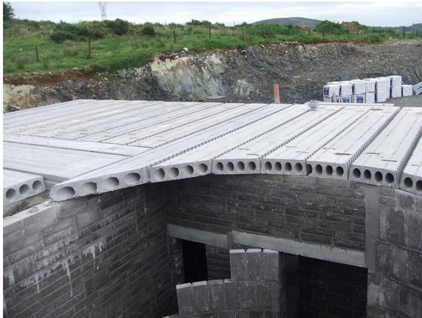
Fig. 8 Hollow core precast concrete slab
