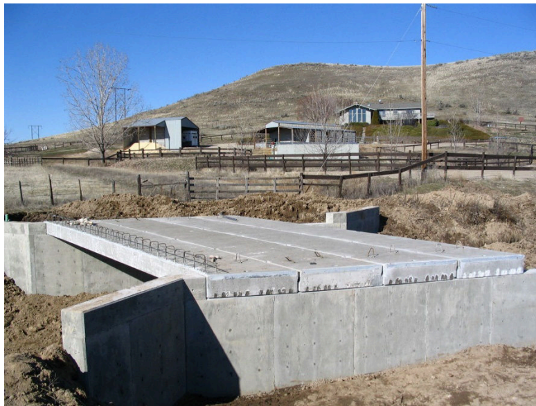
Fig. 12 Precast Solid Deck Bridge made by (Old Castle) comp.
