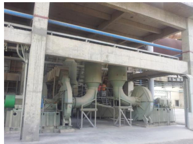
Figure 4 Clinker Crusher and (b) Cooling Fans of Claudius Peter Cooler
