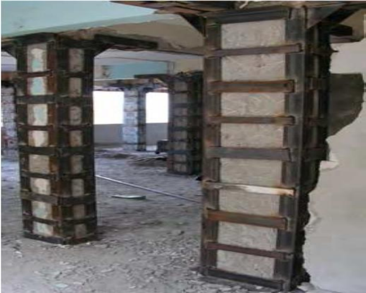
Figure 4 Steel jacketing applied to RC columns
