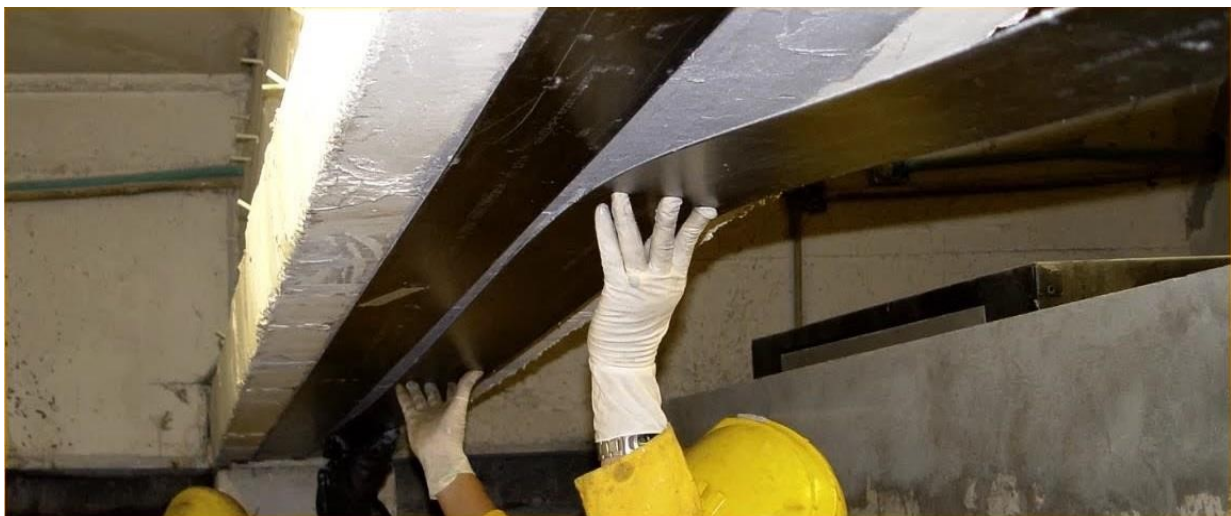
(Figure 7) Flexural strengthening
