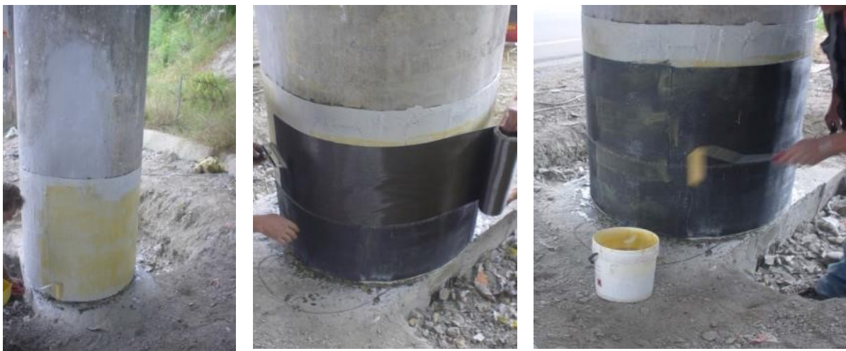
(Figure8) Confinement strengthening
