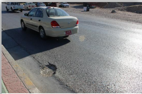
Figure 6. Potholes
