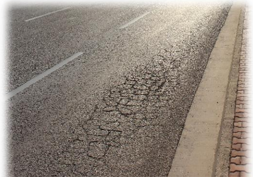
Figure 2. Fatigue Cracking
