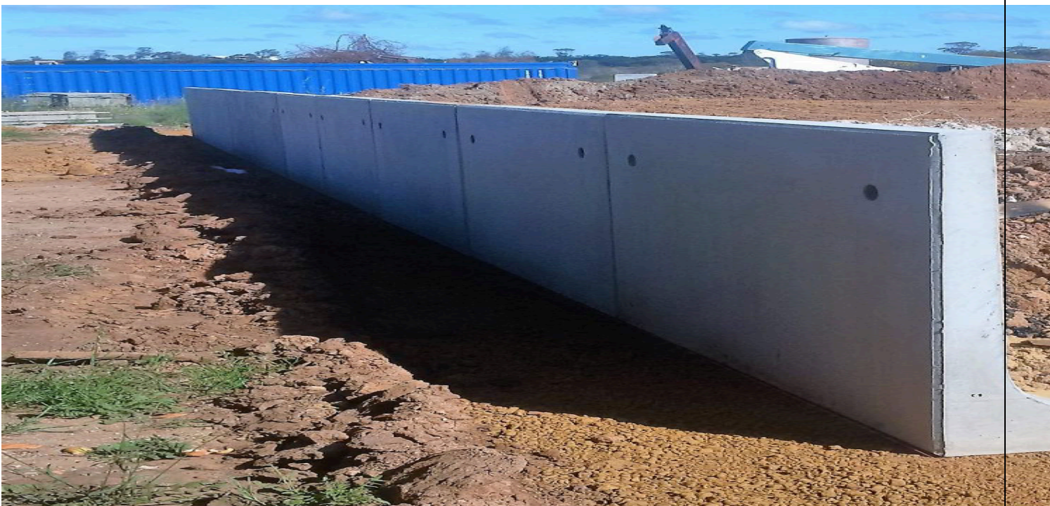
On site of retaining wall construction
