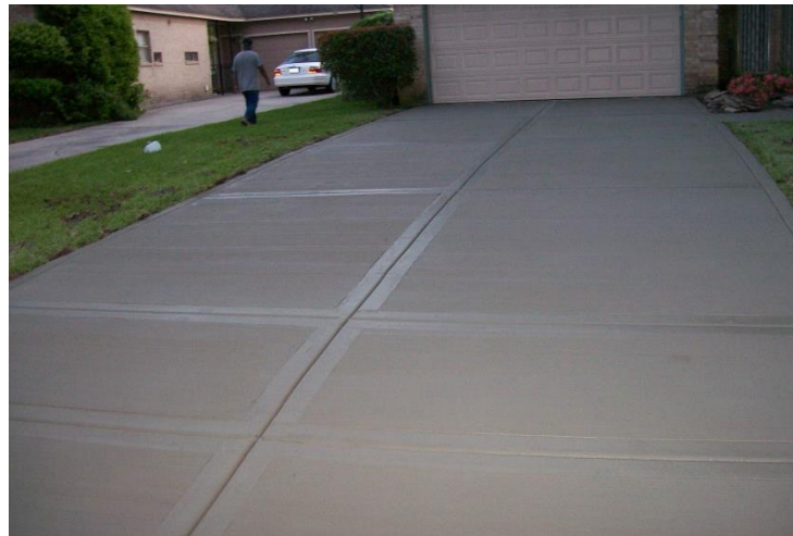
Figure (1): Joints in concrete can serve both to prevent cracking and as a decorative element
