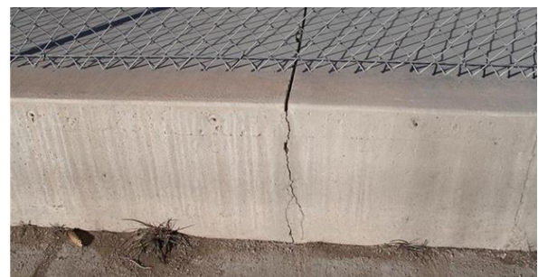
Figure (8) : Slabs crack directly beneath saw cut contraction joints and transfer load between panels by aggregate interlock
