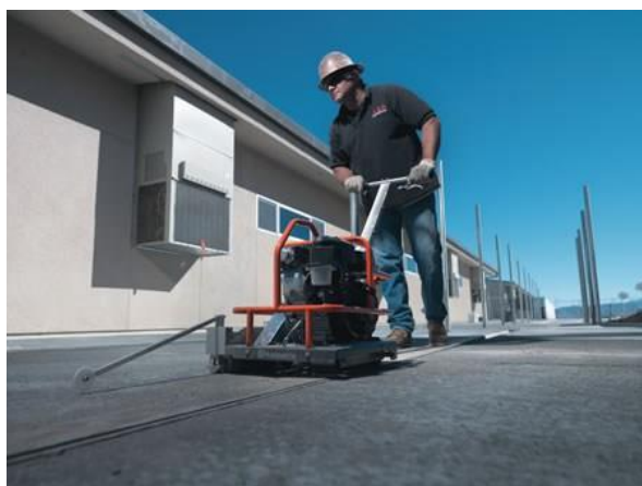
Figure (7) : Early entry saws cut a contraction joint before the concrete has a chance to begin shrinking
