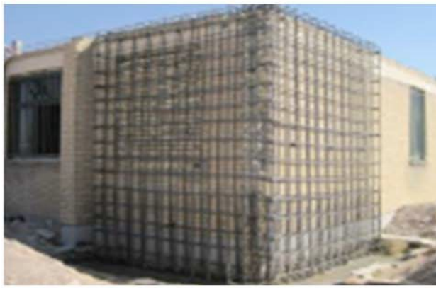
masonry steel mesh outside steel mesh inside
