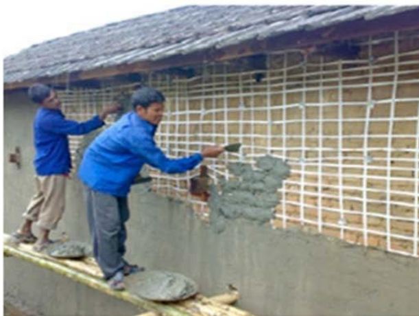
Application of CFRP / GFRP on a building wall
