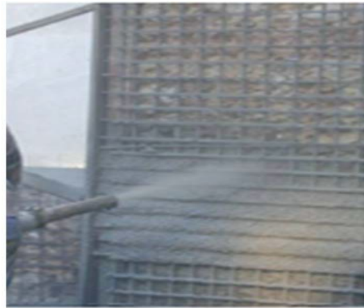
shotcrete over steel mesh
