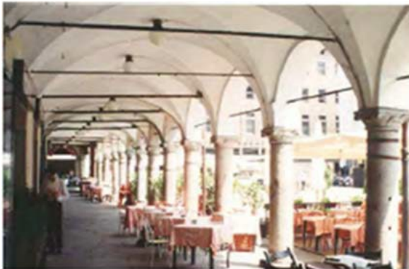
strengthening with tie rods
