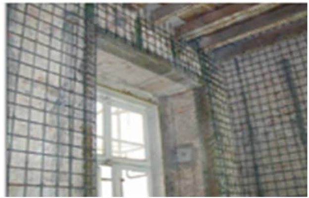
masonry steel mesh outside steel mesh inside
