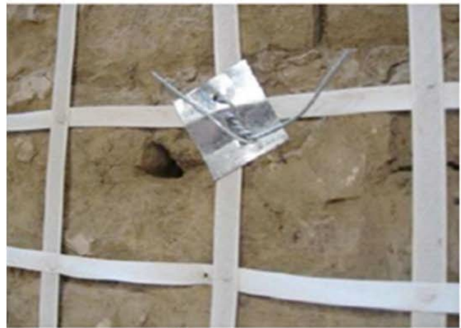
Application of CFRP / GFRP on a building wall
