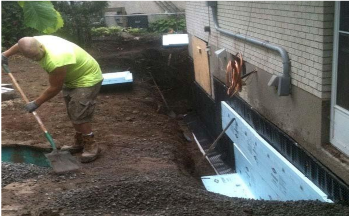
Fig. (4.2) Waterproofing of foundation
