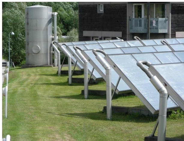
Figure 3: Example of a solar district heating system
