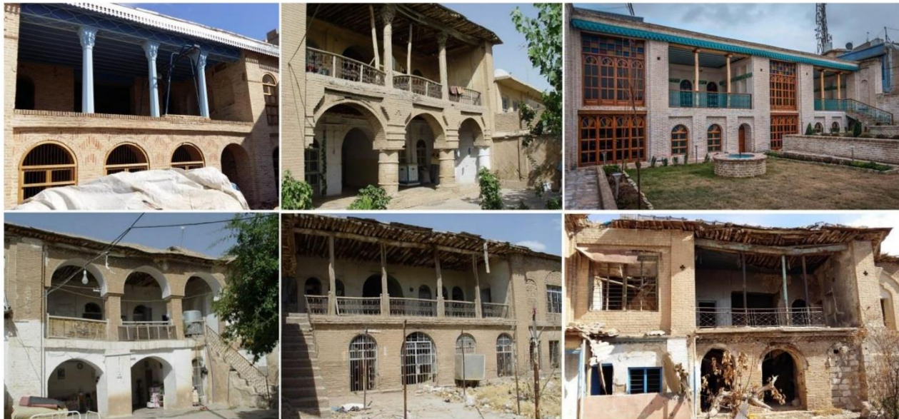
Figure (5) Six examples of traditional houses with iwan in Sulaymaniyah's old town. Source: (Abdulrahman et al., 2019)
