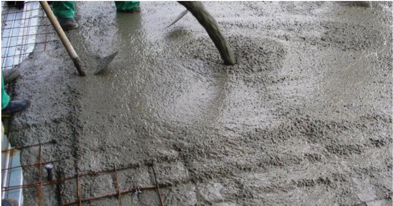
Figure 1 : self compacting concrete
