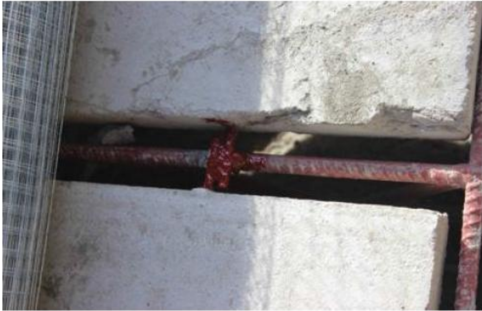
Fig. ٣. ١٥ Re-application of Red Metal Oxide to weld Connections
