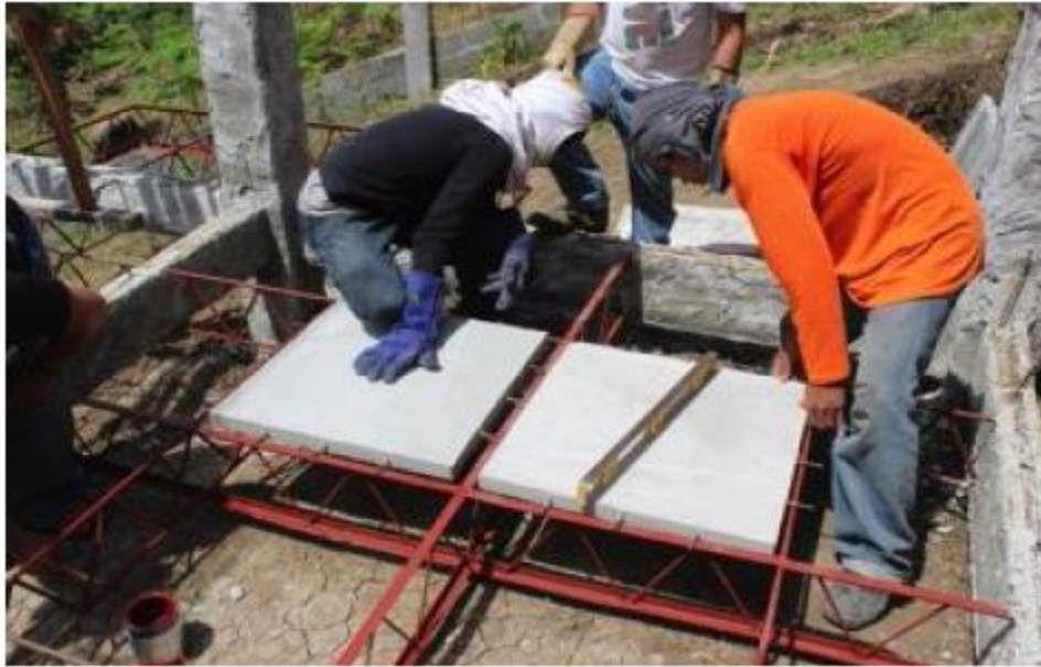
Fig. 3. 13 Installation of another Adjacent Slab
