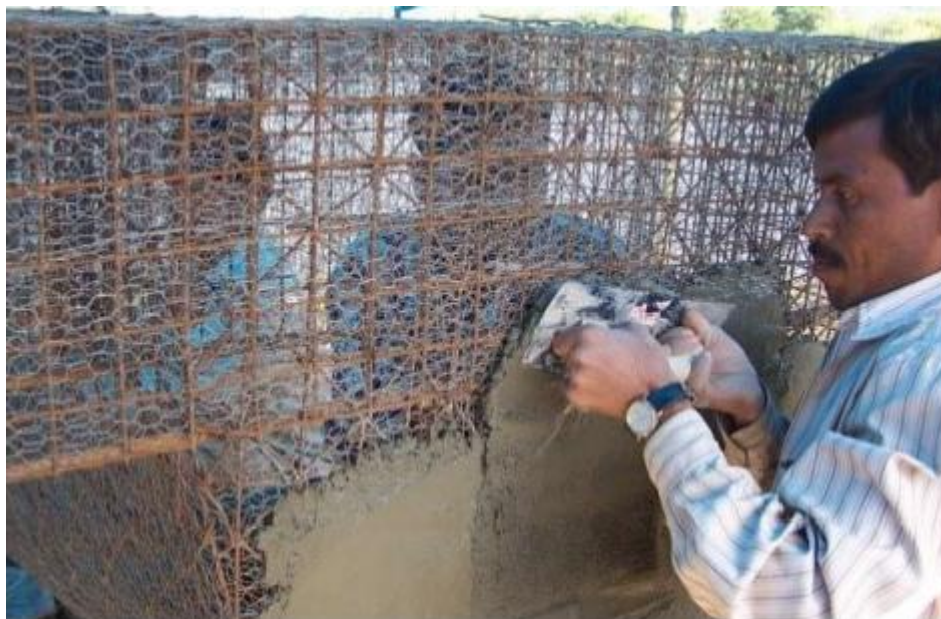
Fig. 1. 7 wall ferrocement construction.
