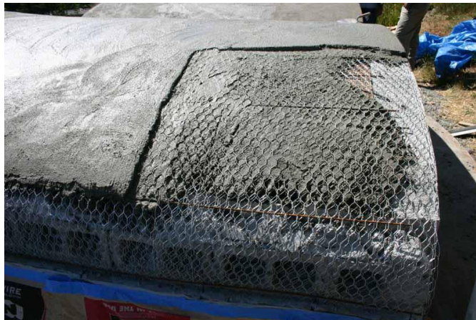
Fig. 1. 1 Ferrocement roof under construction.
