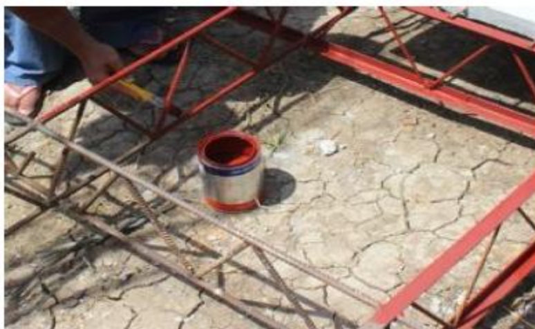
Fig. 3.11 The Application of the Red Metal Oxide to Joists
