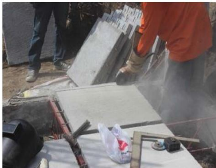
Fig. 3. 14 Trimming of the Slab by using Stone Cutter
