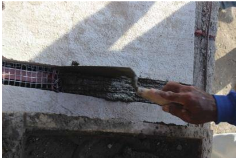
Fig. ٣. ١٦ The Application of the Grout to the Spaces between the Modules
