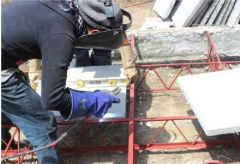
Fig. ۳. ۱۲ Installation of the Modules by Welding
