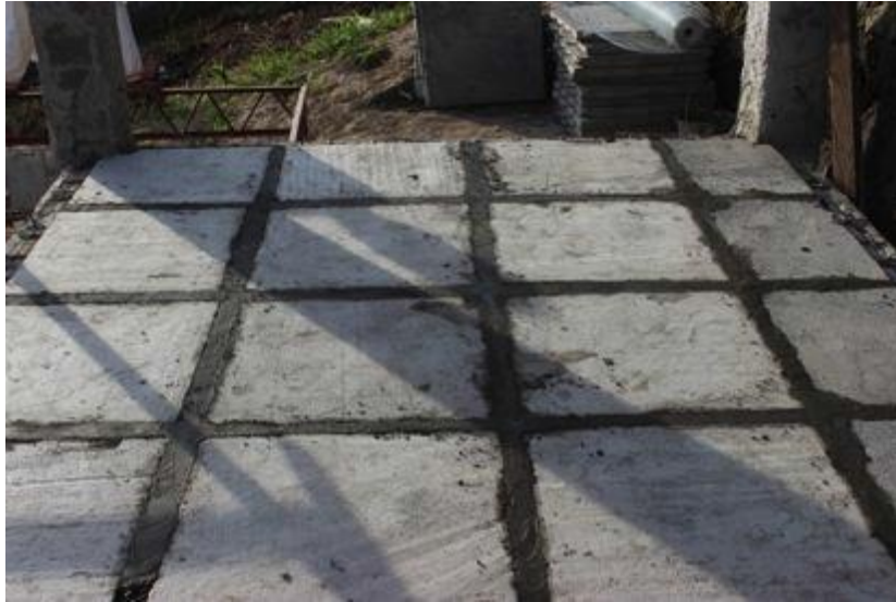
Fig. 3. 14 The Finished System showing Freshly Placed Grout
