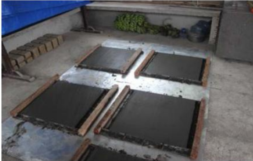
Fig. 3.10 The Molded Prefabricated Slabs Readied for Curing
