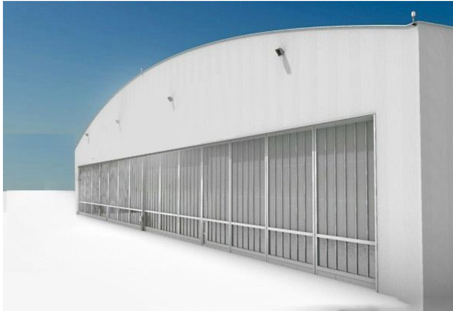
Figure (4) Hangar elevation and main door
