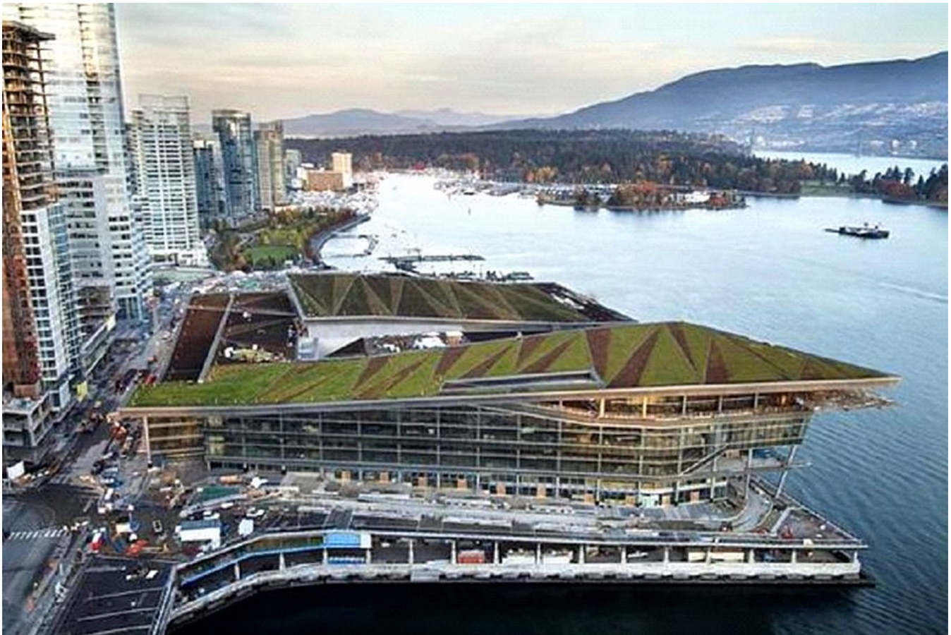
Bird's eye view of the building._@ https://www.greenroofs.com/projects/vancouver-convention-centre-expansion-project
