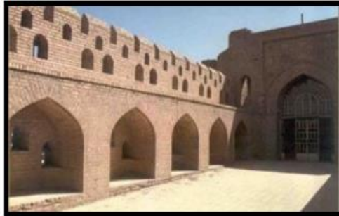
Figure 16: Photo of One Door of Baghdad and Part of Fence [26]
