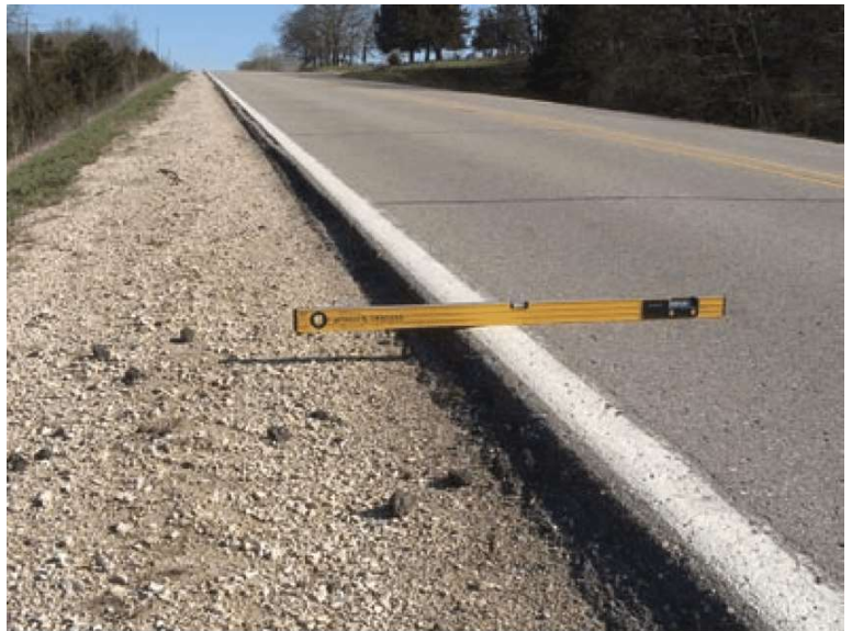
Figure 8: Pavement-Edge Drop-off
