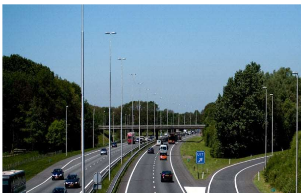
Figure 5: Passive safe columns and sign posts
