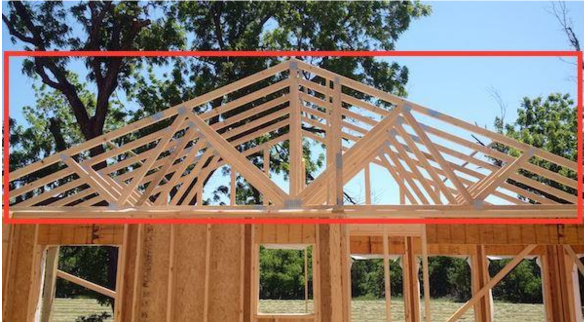
Fig. 6: Truss-framed Construction
