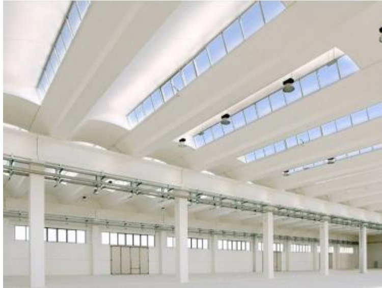
Figure 13 Precast elements of SCC [13]
