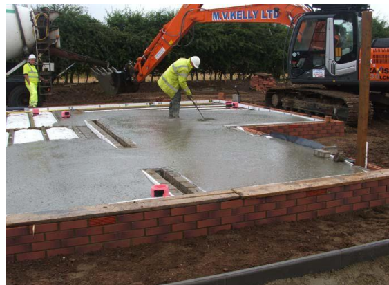
Figure 14 Placing slab of SCC[13]
