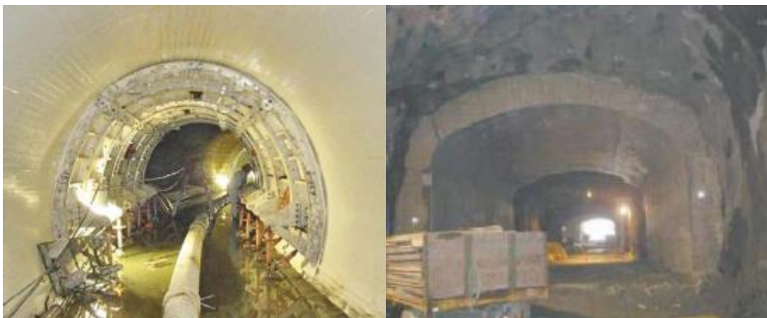
Figure 10 a) Tunnel picture in Los Angeles, USA b) View of the tunnel arch in SWEDEN [10]
