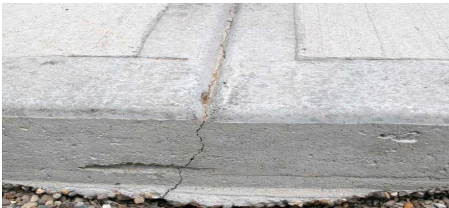
crack at slab penetration Figure ۲
