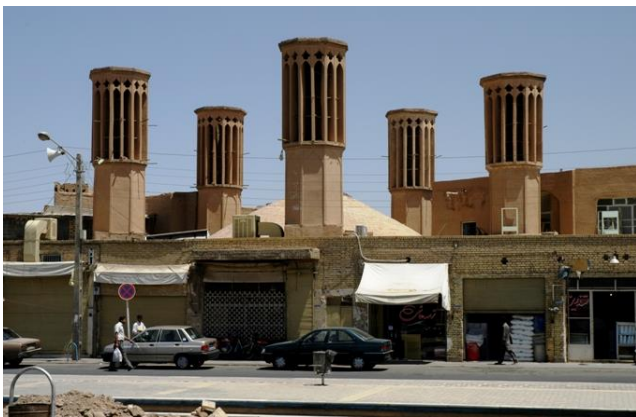
Fig.9 shows wind tower in Yazd, Iran
