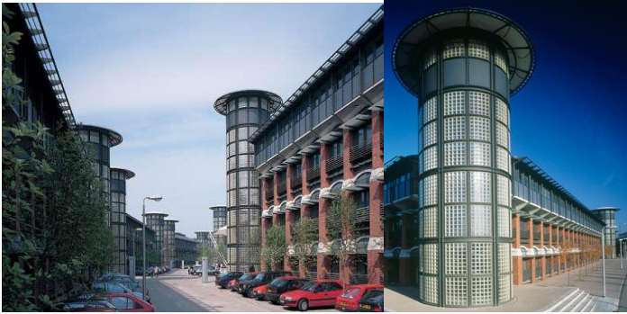
Fig.15 The Inland Revenue Building in Nottingham, designed by Michael Hopkins and partners [12].
