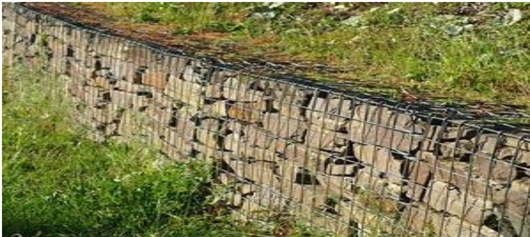
Figuer 9. Gabion wall Retaining Wall
