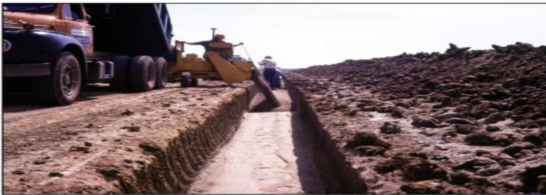
Figure 7-6. Trenching method – backfilling trench.
