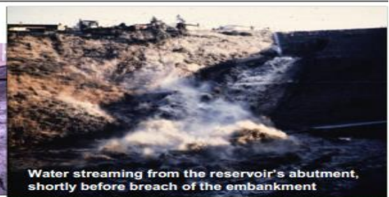
Piping occurred along a branch of the Newport-Inglewood fault, shown below
