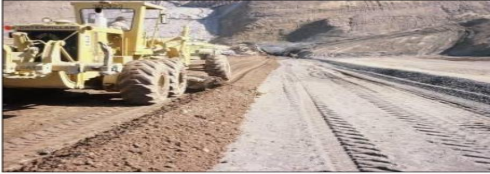
Figure 7-3. Windrowing impervious material adjacent to a filter/drain.
