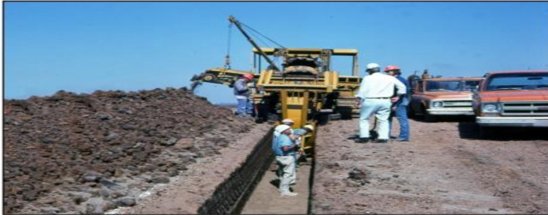
Figure 7-5. Trenching method – excavating trench.
