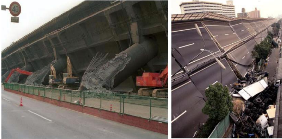
Single Pier- Inadequate ductility
