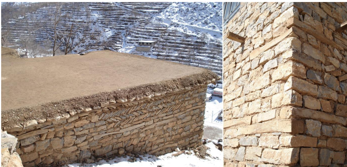
Figure 4: building construction components and materials in Tawela vernacular house, (photos: Author, 2007)
