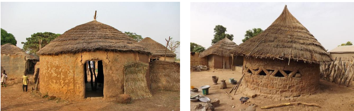
Fig (3) Typical Adobe building in Ghana. Source: reference (Agyekum et al., n.d.) [2]
