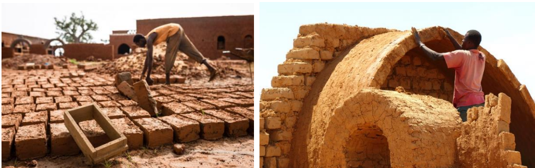
Figure (8) A Typical Vaulted brick building in Ghana. Source: reference (Agyekum et al., n.d.)
