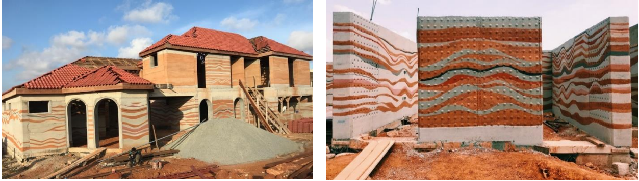
Fig (7) A Typical Rammed earth building in Ghana. Source: reference (Agyekum et al., n.d.)
