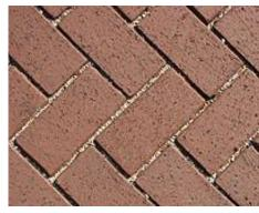
2-Pervious pavers: Allow drainage through the pavers themselves.
