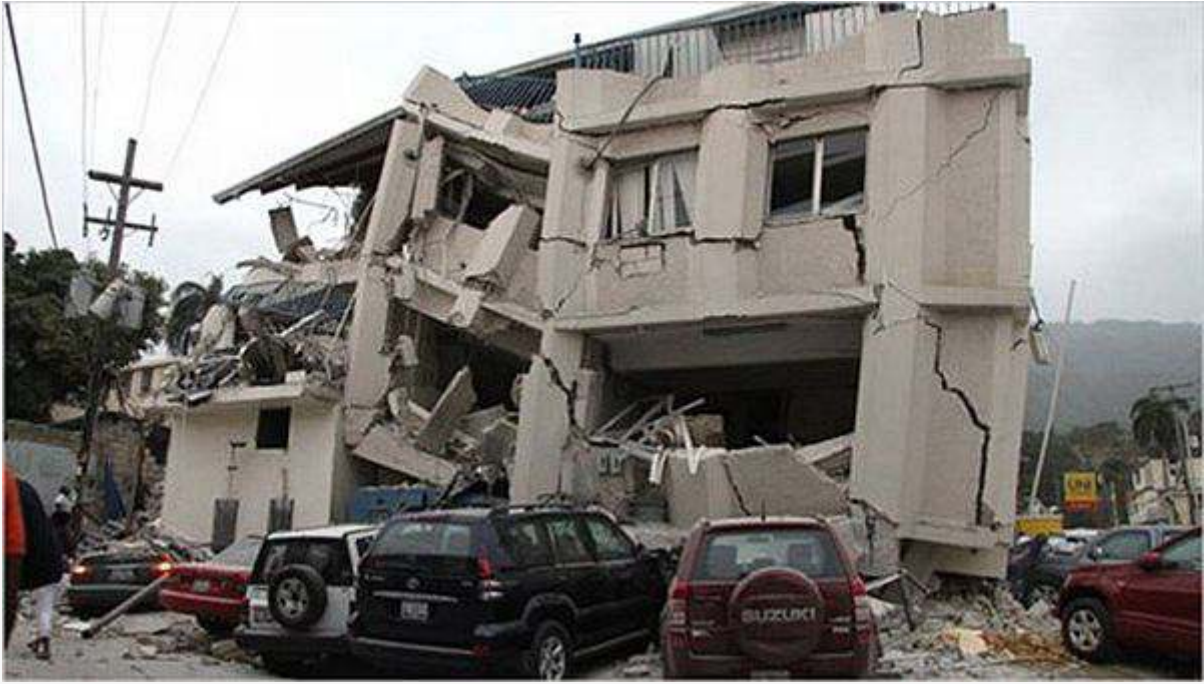
Haiti Earthquake Damage 2010
