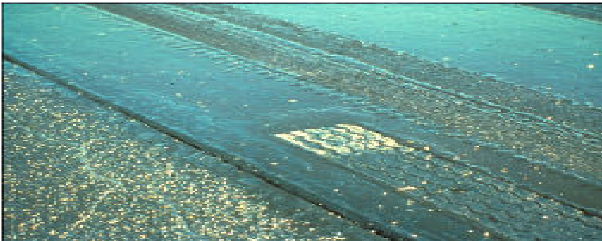
Figure 3-2-17. Incorrect Tack Coats
