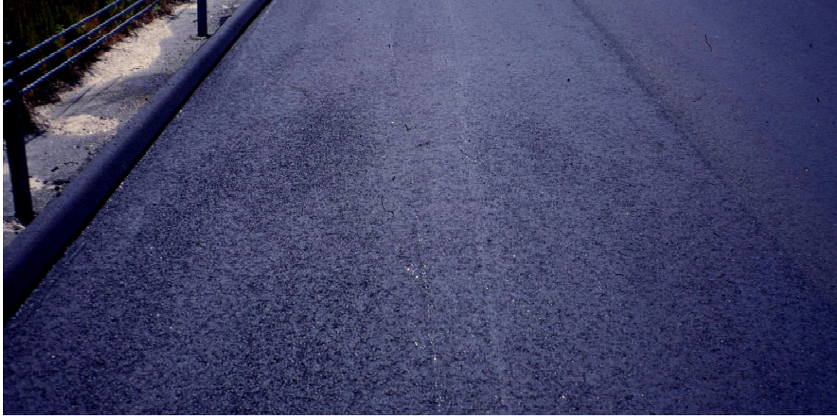
Figure 3-4-11. End of Truck Segregation
