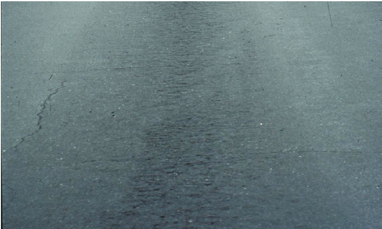
Figure ϣ-ϣ-Ϛ. Centerline Segregation
