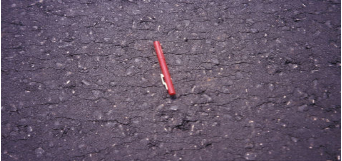
Figure 3-1. Checking Under Roller
