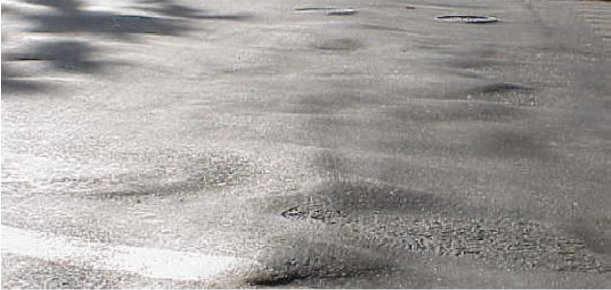
Figure 2-9-8. Unstable HMA
