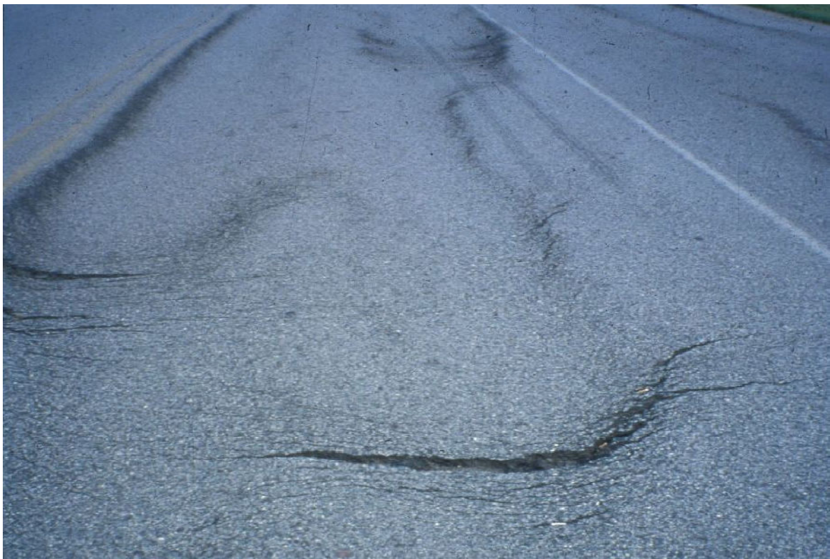
Figure ϒ-ϒ. Mat Tearing Full Width
