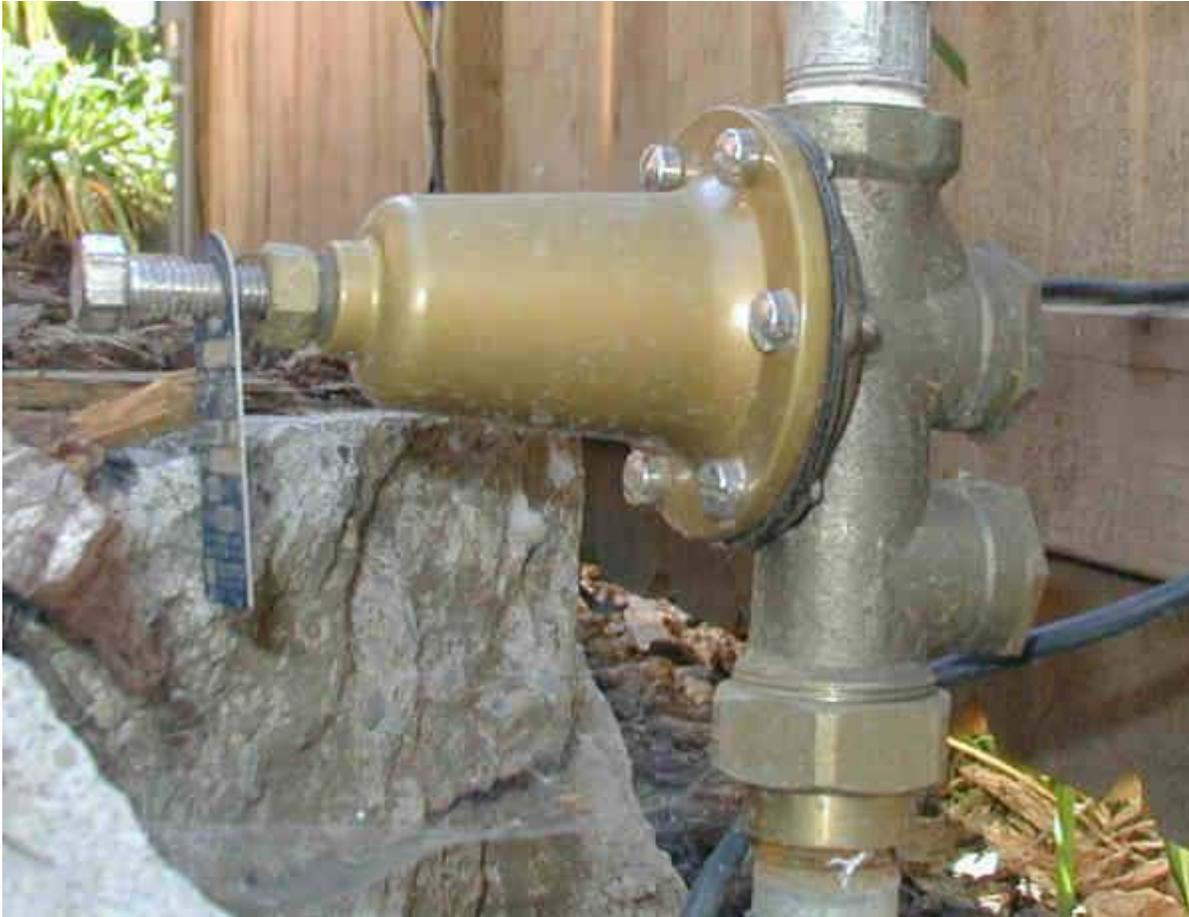
**Pressure Reducing Valve/ Pressure Regulating Valve/ Pressure Regulator**
