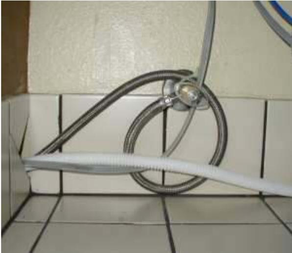
**Typical dishwasher shut-off valve under a kitchen sink. The silver tube looped around the valve is the water supply to the dishwasher. Gray is the dishwasher power cord. White pipe is the dishwasher drain pipe.**
