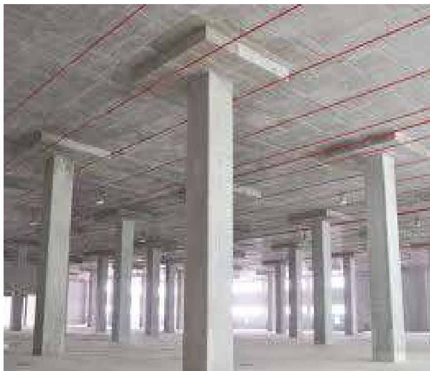
Flat slab with drop panels
