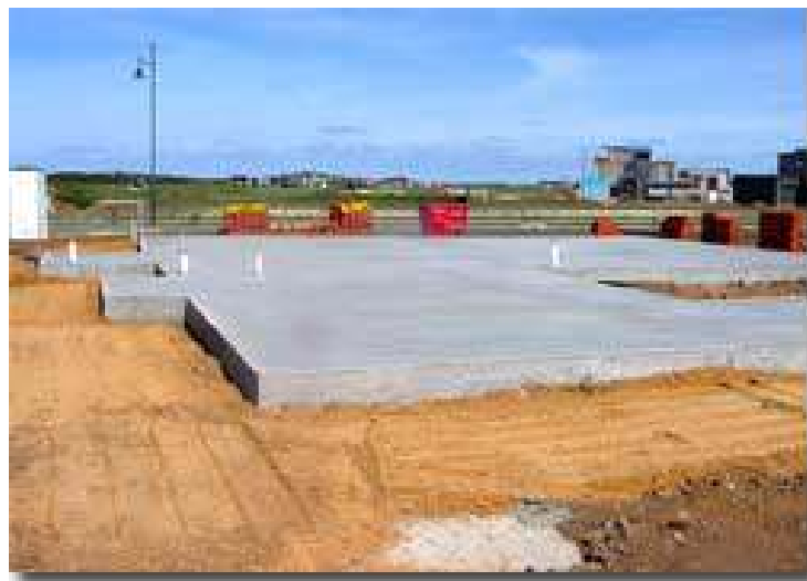
Stiffened raft slab
