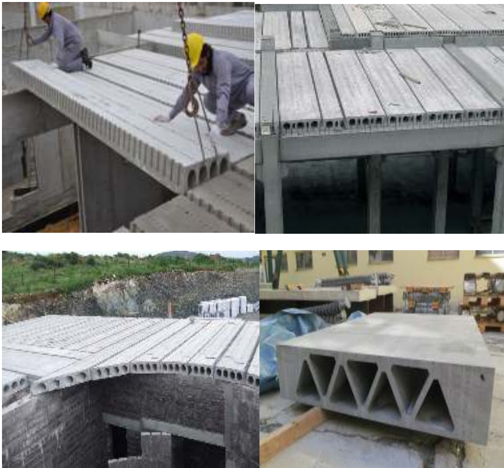
Hollow core slab
