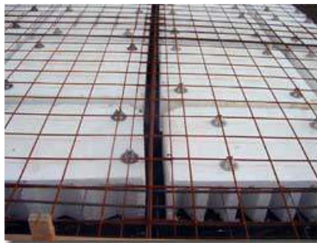
Polystyrene void forms below reinforcement.
