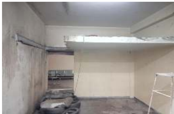
Low roof slab
