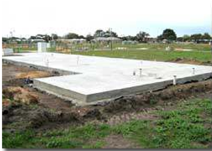
Concrete slab on the ground
