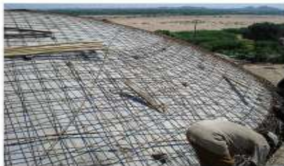
Dome Slab laid on Conventional Slab
