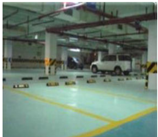
Figure 4 - (a) Self-leveling mortar as floor covering Figure 5 - (b) Self-leveling mortar cover with epoxy
