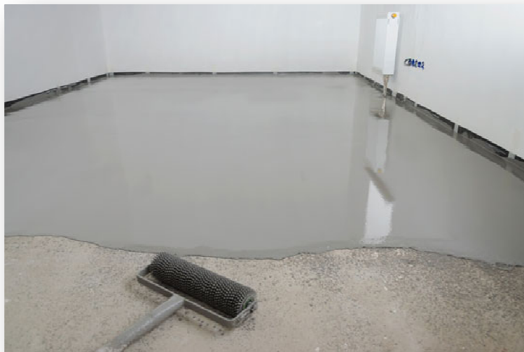
Figure 1: Examples of the use of self-leveling Concrete
