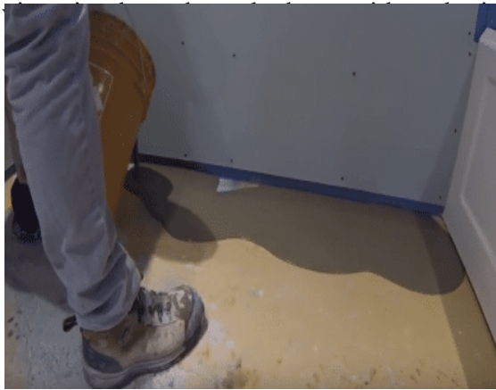
Figure 6 - Pouring SLC Mix Figure 7 - Spreading SLC with a Gauge Rake
