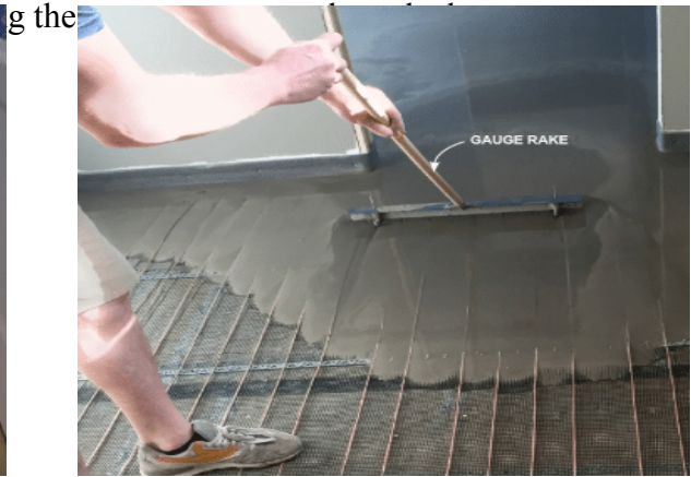
Figure 6 - Pouring SLC Mix Figure 7 - Spreading SLC with a Gauge Rake
