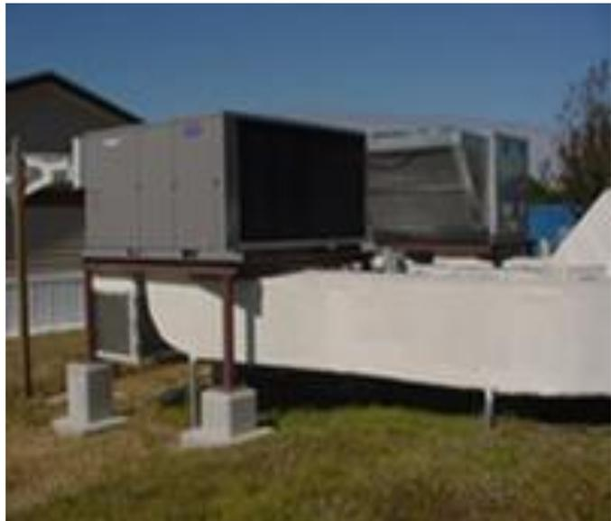
A packaged system is a single unit combining all the components described in the split system. Since the unit is a package, it must be placed outside the building and indoor air is “ducted” from the building to the packaged system and back through an air distribution system. These units typically have SEER rating from 10 to 18. If heating is required, an alternate method of heating the interior of the building must be used, usually in the form of electric or gas heating.
