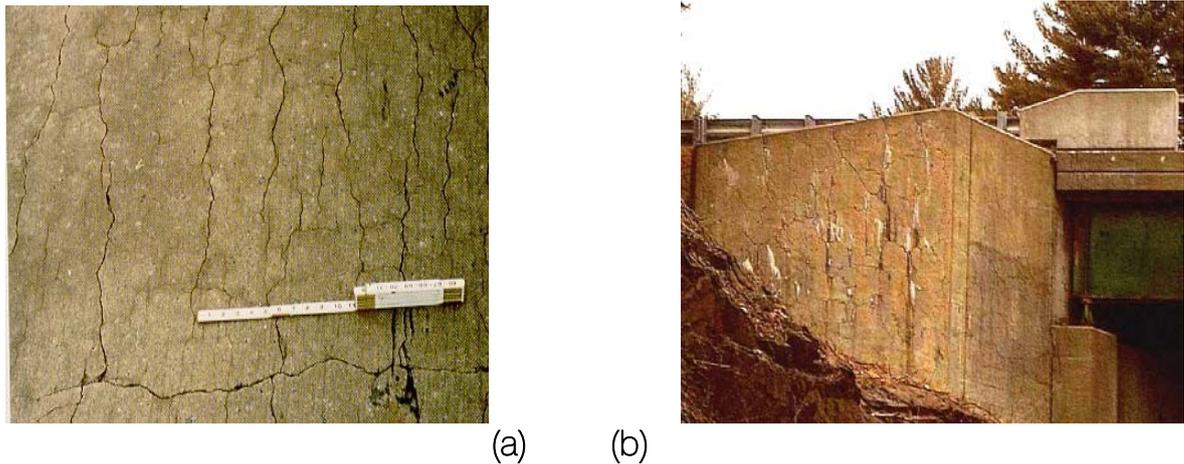
FIGURE 12 Alkali aggregate reaction: (a) a 355-mm (14-in.) airport pavement at Pease International Airport, Portsmouth, New Hampshire, and (b) a bridge end wall on I-95 in Kittery, Maine.
