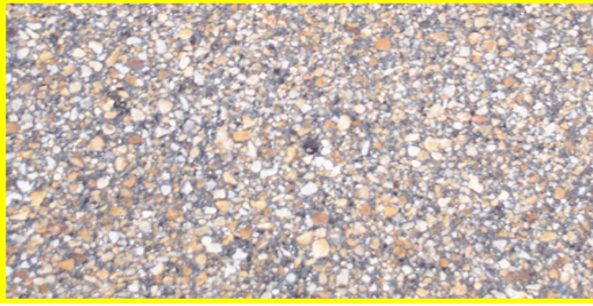
Low: Binders and fines have eroded away
