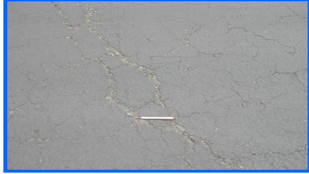
Low: Binders and fines have eroded away
