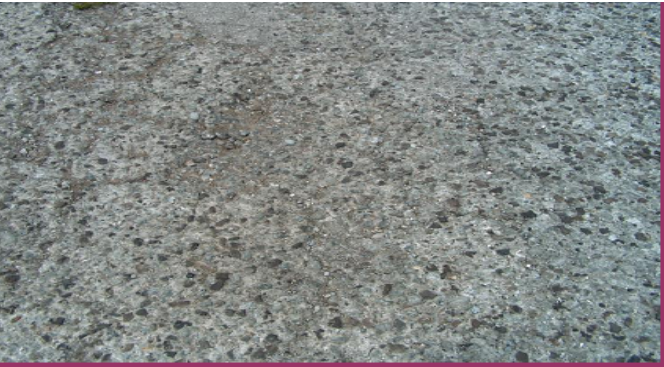
High: Nearly all the surface aggregate has eroded away.
