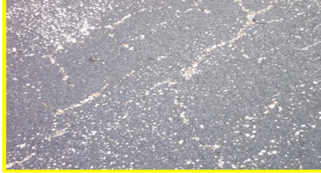
Medium: nearly 50% of surface aggregate has eroded away.
