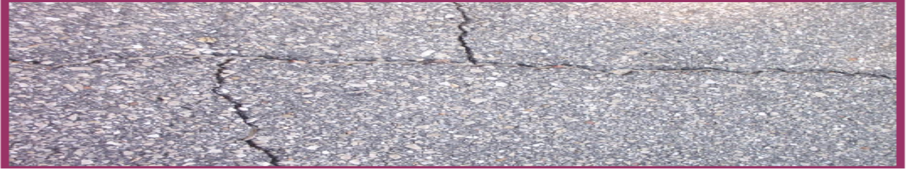
High: Combination of both longitudinal and transverse
