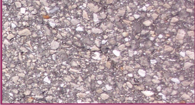
Medium: nearly 50% of surface aggregate has eroded away.
