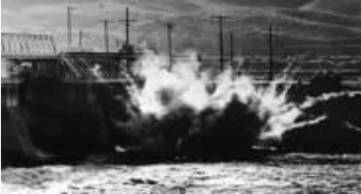
Figure 26. Dynamite is used for removing the Lewiston Dam ([15])
