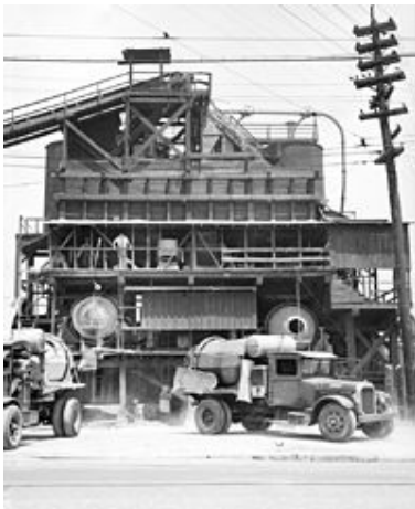
Concrete mixing plant in Birmingham, Alabama in 1936
