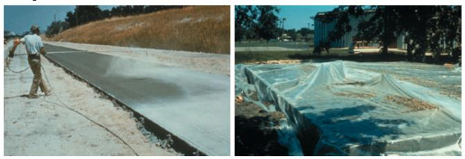
Liquid membrane-forming compounds sprayed onto the surface are effective, economical moisture barriers for moist-curing concrete.
