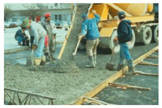
then leveled and worked together; nor should the concrete be deposited in large piles and moved horizontally into final position.
