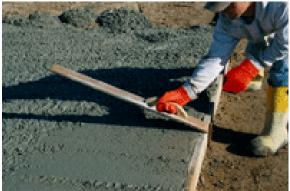
of cutting off excess concrete to bring the top surface of the slab to proper grade. A straight edge is moved across the concrete with a sawing motion and advanced forward a short distance with each movement.
