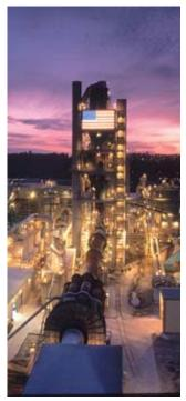
final grinding process to regulate the setting time of the concrete. Lime and silica make up about 85% of the mass. Common among the materials used in its manufacture are limestone, shells, and chalk or marl combined with shale,
