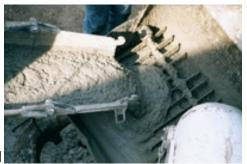
loss in workability. As a result of the slump loss, superplasticizers are usually added to concrete at the jobsite.
