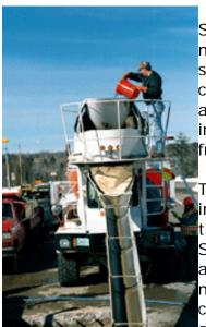
Successful use of admixtures depends on the use of appropriate methods of batching and concreting. Most admixtures are supplied in ready-to-use liquid form and are added to the concrete at the plant or at the jobsite. Certain admixtures, such as pigments, expansive agents, and pumping aids are used only in extremely small amounts and are usually batched by hand from premeasured containers.
