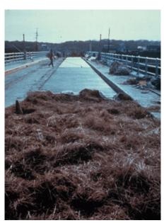
Burlap kept saturated with water is an effective medium for moist-curing concrete. Straw or hay is still used to insulate fresh concrete in freezing weather.
